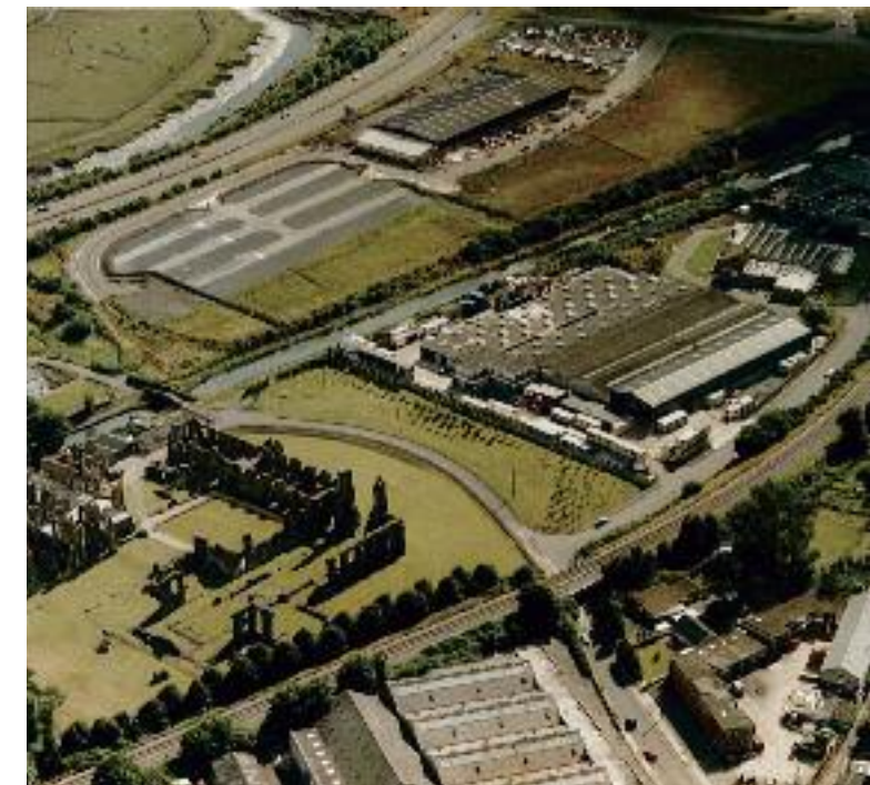
An aerial view of the site of the Neath factory, acquired by Wernick in 1989.
