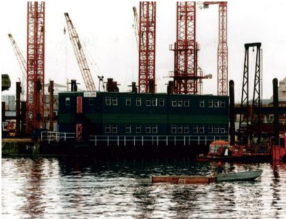
This floating base camp was supplied by Wernick in 1988 for the London Docklands development.
