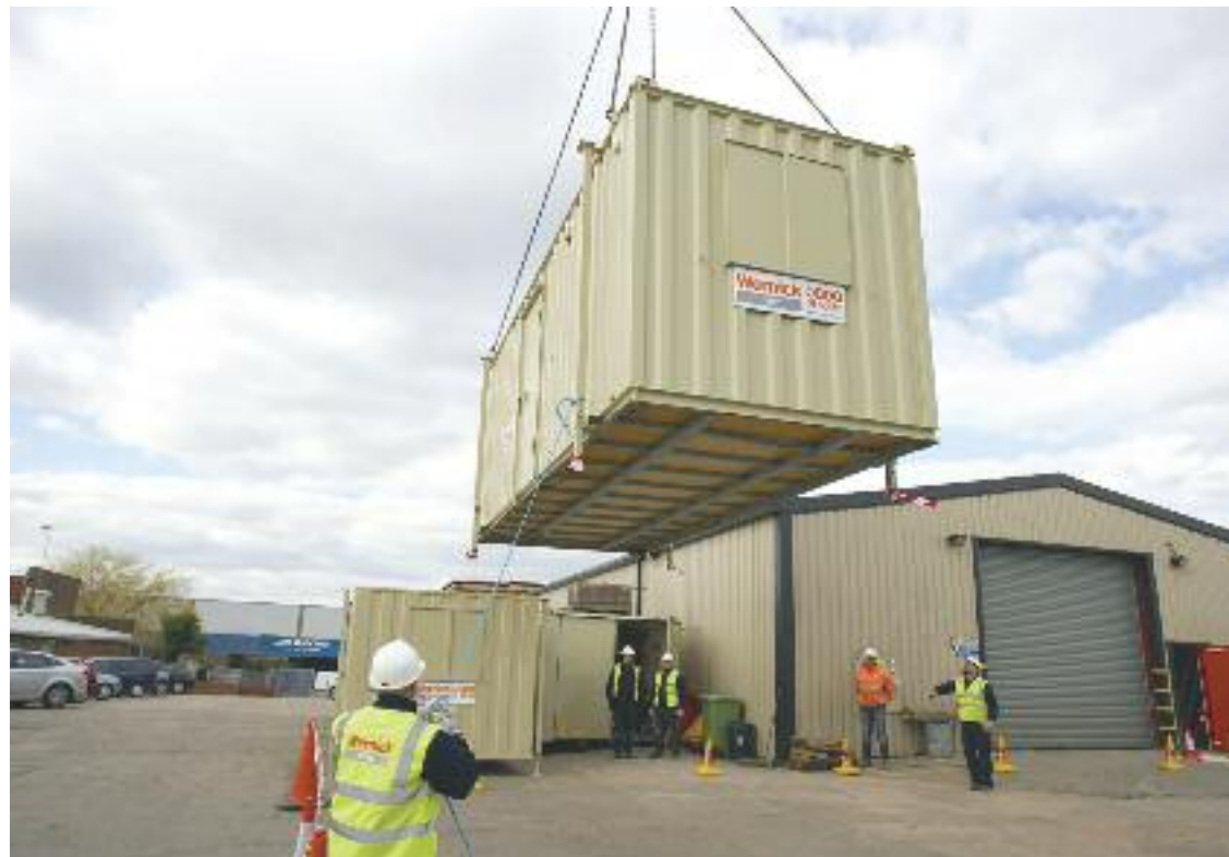
A Wernick Anti-Vandal unit being craned into position at a Wernick depot.
